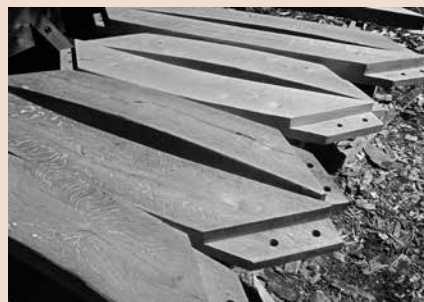
The diagonal braces are matching pairs cut from naturally curved logs. They are placed so that the grain pattern of one brace is a mirror image of the opposing brace.
