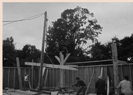
The diagonal braces are matching pairs cut from naturally curved logs. They are placed so that the grain pattern of one brace is a mirror image of the opposing brace.
