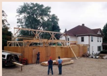
At the end of the day, the walls are buttoned up by the general contractors (Emerson Brothers). The 50' ridge beam will be supported at its ends by the gable stud walls. Note the gin pole on the truck roof at left.
