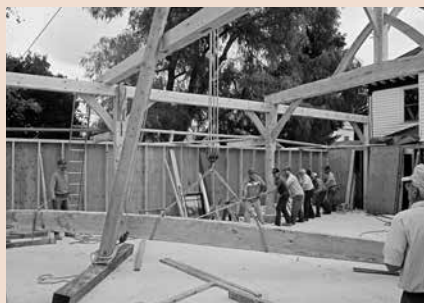
One of the big tie beams is being raised by six lodge brethren. The six-part block and tackle multiplies their force by six times. Note the pulley at the base of the gin pole that changes the direction of pull to horizontal.
