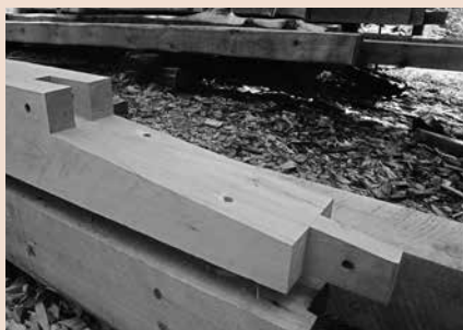
The 50 foot purlin plates and ridge beam are made of two shorter timbers "scarfed" together. This scarf utilizes two mortise and tenon joints and four pins.
